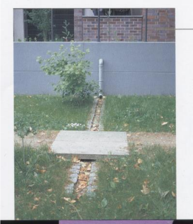
Figure 2: Drainage of rock pit through sidewalk channel
