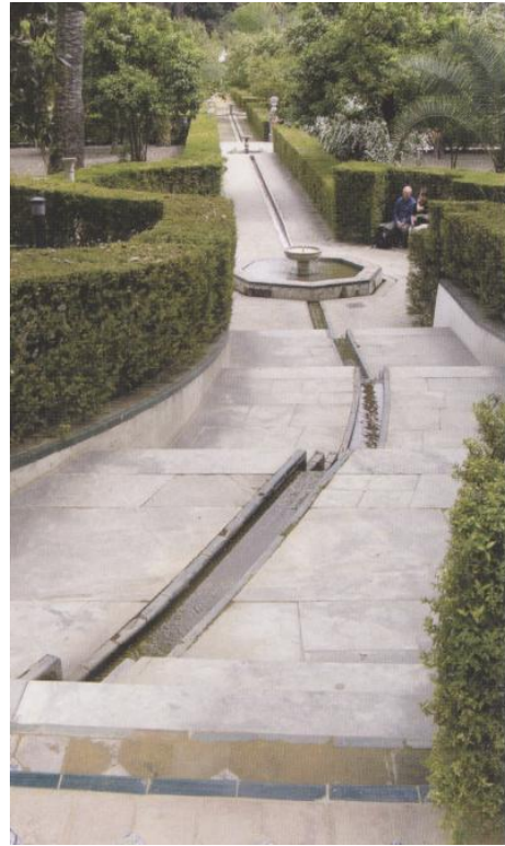
Figure 12: Integrated watercourse with elevation changes
