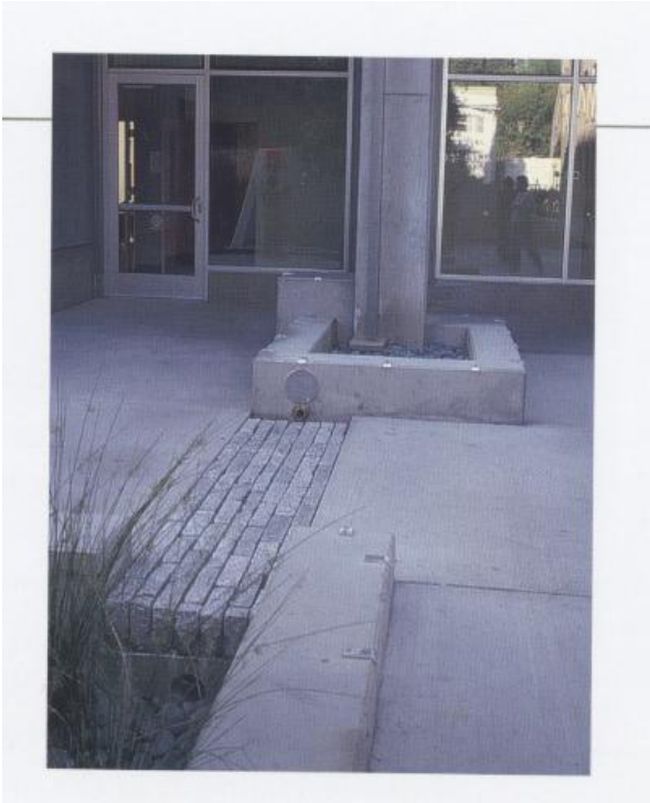
Figure 2: Drainage of rock pit through sidewalk channel
