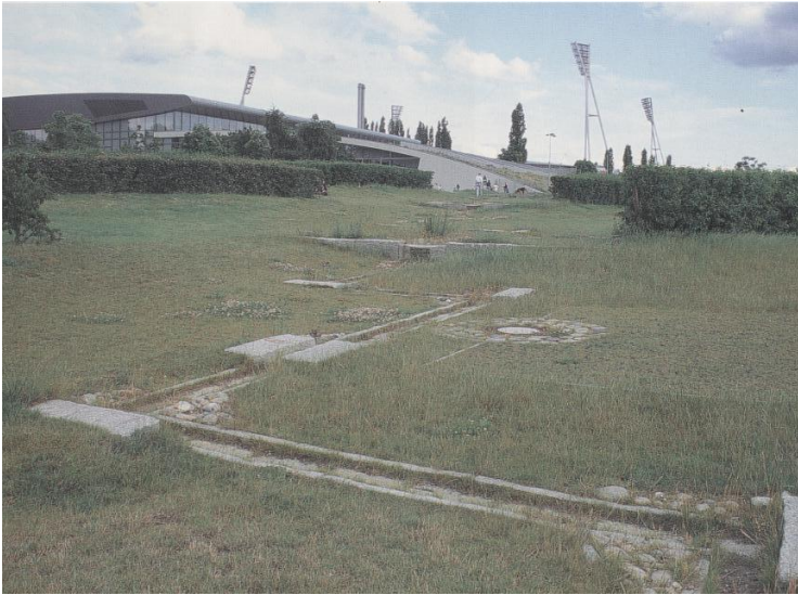
Figure 11: Open drainage channels
