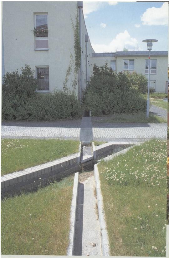
Figure 5: Roof drainage via drainage channels
